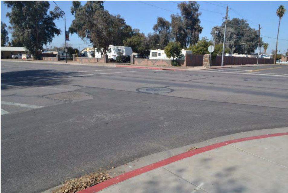
Looking northwest from southeast corner of intersection 2.
