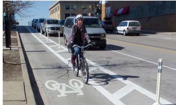
Protected bike lane with pavement marking buffer and vertical delineators
