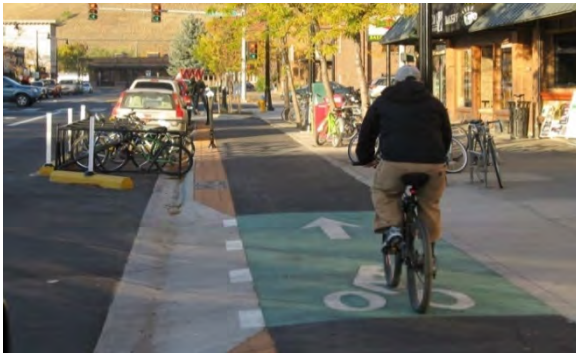
Protected bike lane with elevated lane
