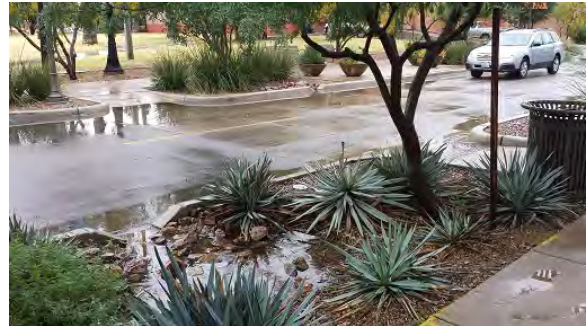
Example of bioinfiltration planter: Stormwater entering and infiltrating
