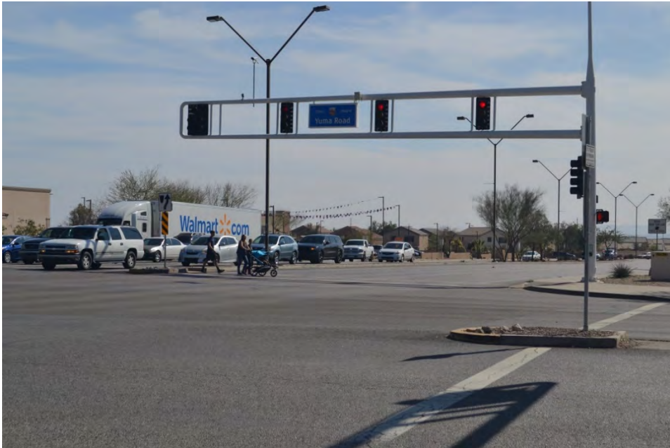
Looking south from northwest corner of intersection 1.
