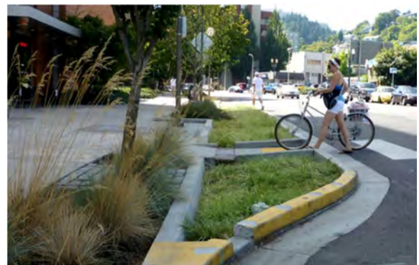
Bulb-out/Curb Extension with stormwater infiltration
