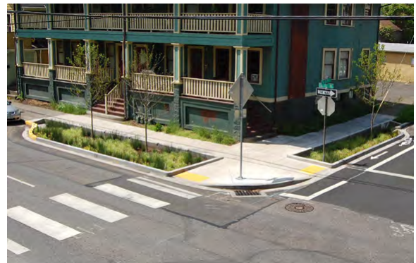
Bulb-out/Curb Extension with stormwater infiltration
