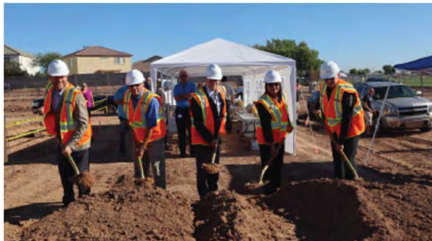
Police Evidence & Training Center Phase I Groundbreaking, Fall 2019
