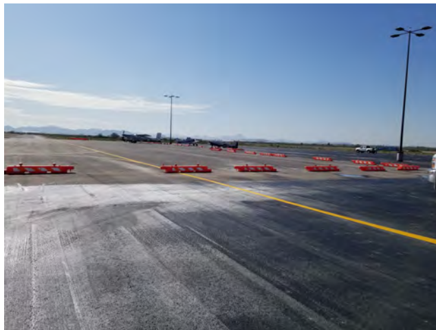
Airport Taxiway & Southern Apron Reconstruction, Winter 2019
