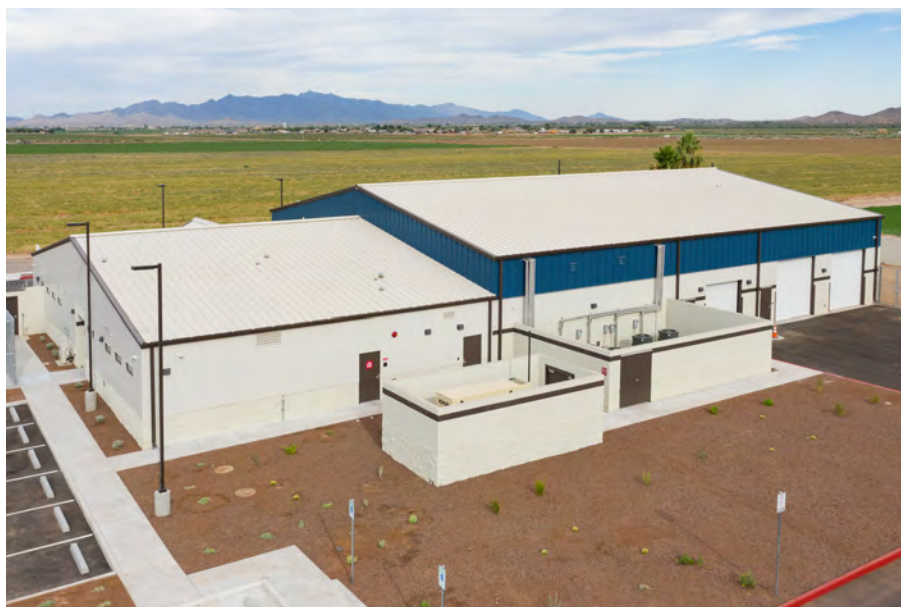
Police Evidence & Training Facility Phase I, Completed Summer 2020
