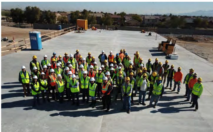
Broadway Road Water Campus pre-topping off reservoir tour, January 2020
