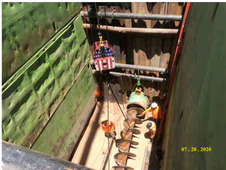
A look inside the North Miller Trunk Sewer Project, Summer 2020
